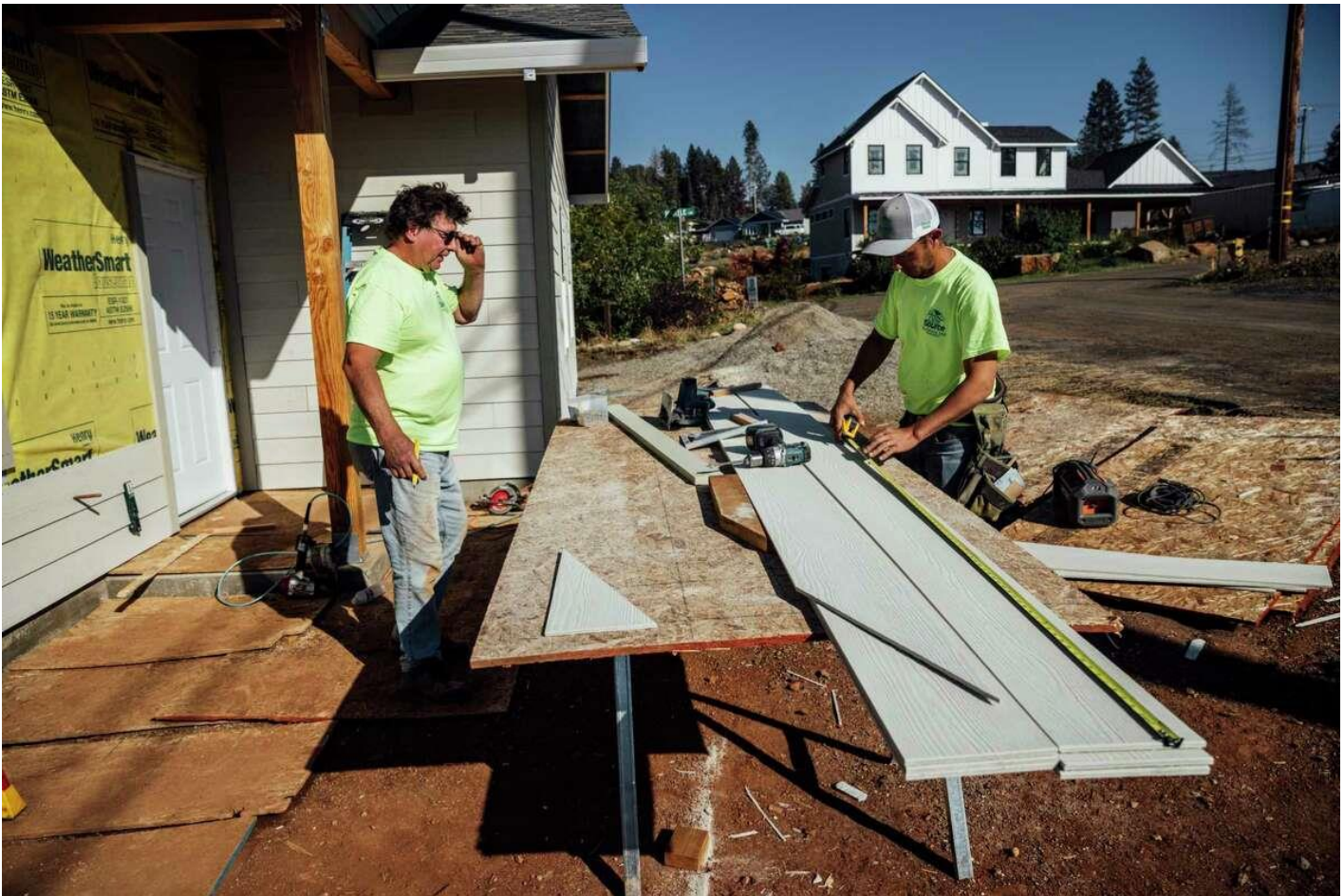
Neville Smith, left, and Michael Delarosa work to add siding to a nearly finished home in Paradise. Stephen Lam/The Chronicle
